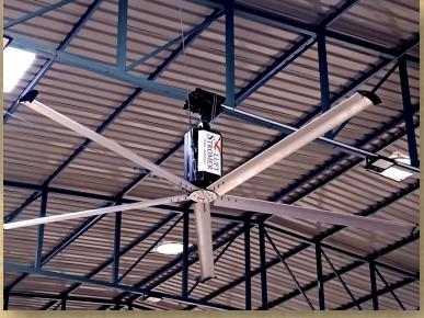
LUFT STROMER HVLS gearless fans use Sophisticated PMSM (Permanent Magnet Synchronous Motor) which has low torque repulsion. PMSM Gearless HVLS fans have better and smooth torque with higher efficiency and extremely low noise compared to the geared fans.
